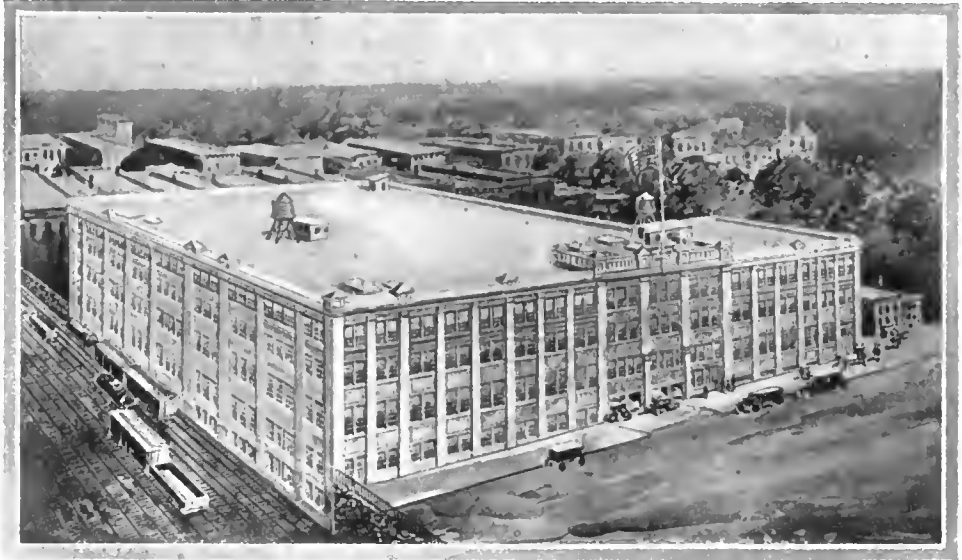
The new garage being built by the Hudson Motor Car Co. of New York
